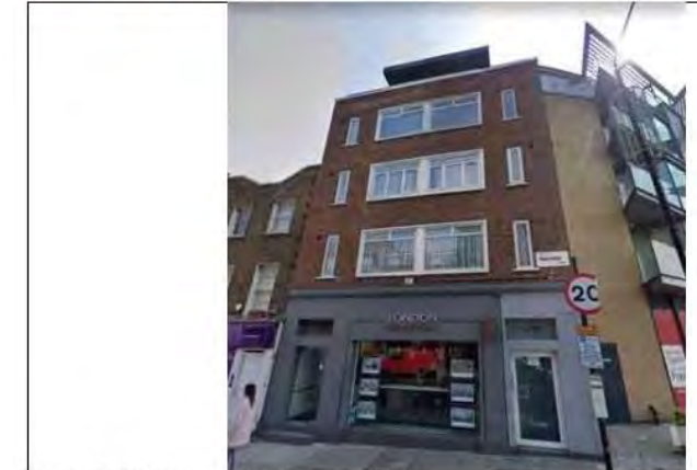
Figure 3 - SCSMW_15785: North-West elevation (Google Maps)
