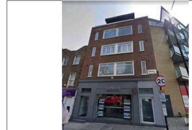
Figure 3 - SCSMW_15785: North-West elevation (Google Maps)
